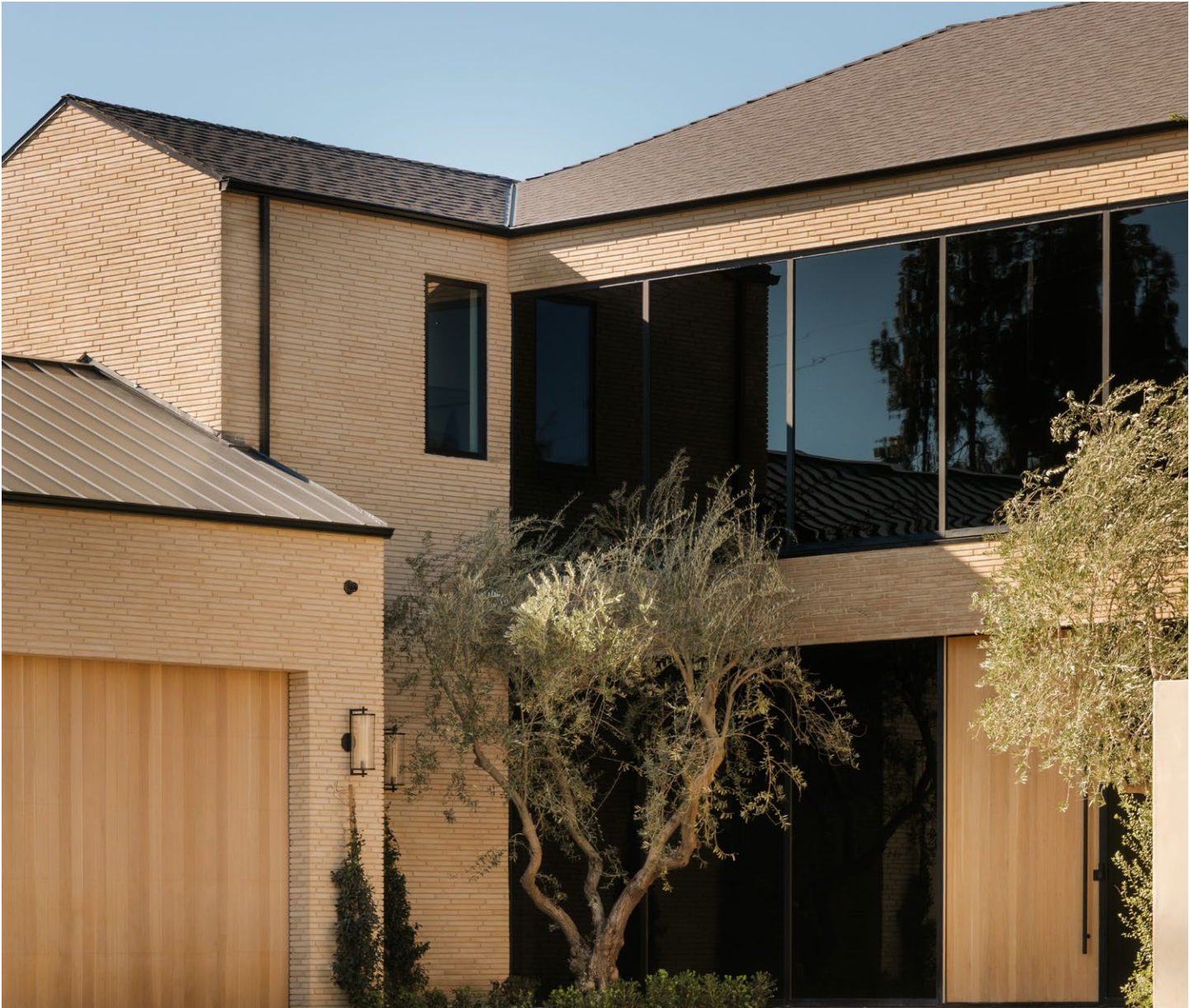
SANDBLUFF Novarra Brick Design: Sophea Interior Design Builder: Pacific Suburb
